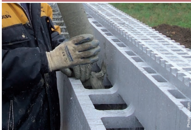
Wall filled up with silo technology or concrete skips
